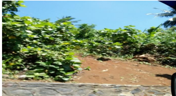
Figure 3. Landslide on a gentle slope
